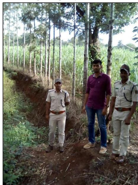
Photo 19: Elephant proof trench, Chikkamagaluru range, Chikkamagalur division & circle Breached and ineffective
