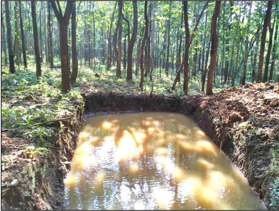
Photo 5: Percolation pit, Batragadde plantation, Aldur range, Chikkamagalur division and circle Appropriate site, good quality, very effective
