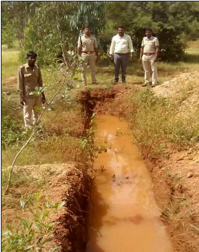
Photo 6: Percolation trench, Gudagur plantation, Ranebennur range, Haveri division Appropriate site, stabilised bunds with vegetation, effective work
