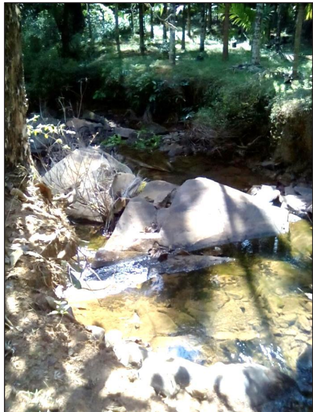
Photo 21: Gully checks, Gerusoppa range, Honnavar division, Uttara Kannada circle Breached and ineffective
