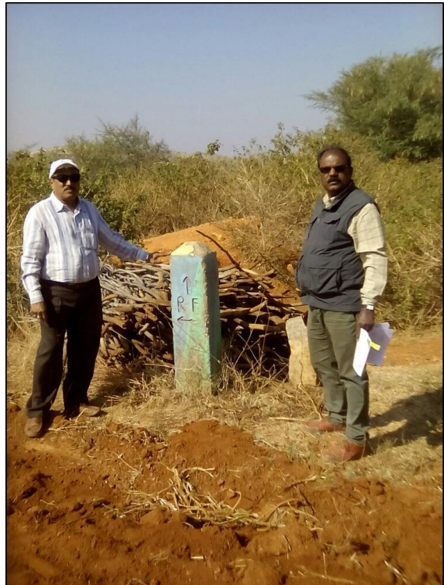
Photo 15: Sunkadakallu Reserve Forest, Kudligi range, Ballari division & circle Durable reinforced cement concrete structure for boundary marking
