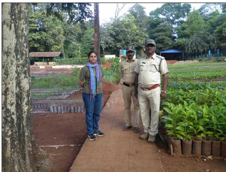
Photo 27: Cement concrete pathway, Idagungi range, Yellapur division, Uttara Kannada circle Well laid out and used everyday
